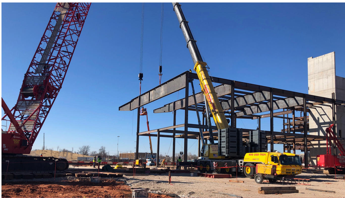
After steel trade staffing complications as a result of COVID-19, Flintco's sister-company, Kienlen, kept the project on-schedule by bringing a team on-site to complete a portion of the massive steel package at the Oklahoma City Convention Center.
