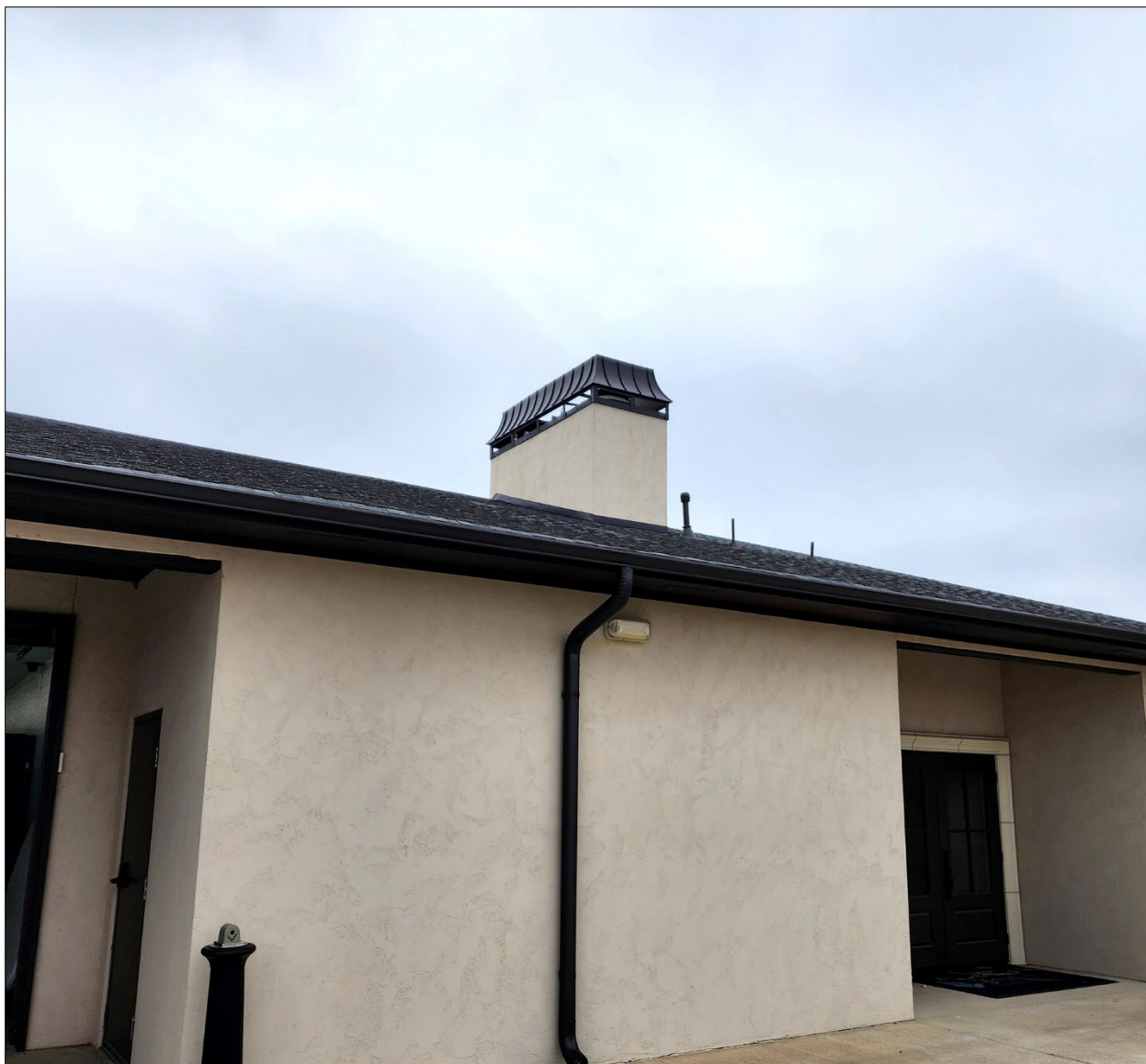
Exhibit 4: Exhaust chimney during cremation process
